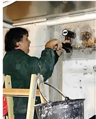
Dubious beam being tested for strength, Denmark
